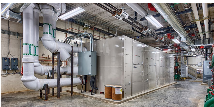
Top: Schematic of the geothermal system in DesignBuilder. Center: The borefield under construction. Bottom: Moduclar heat recovery chiller
