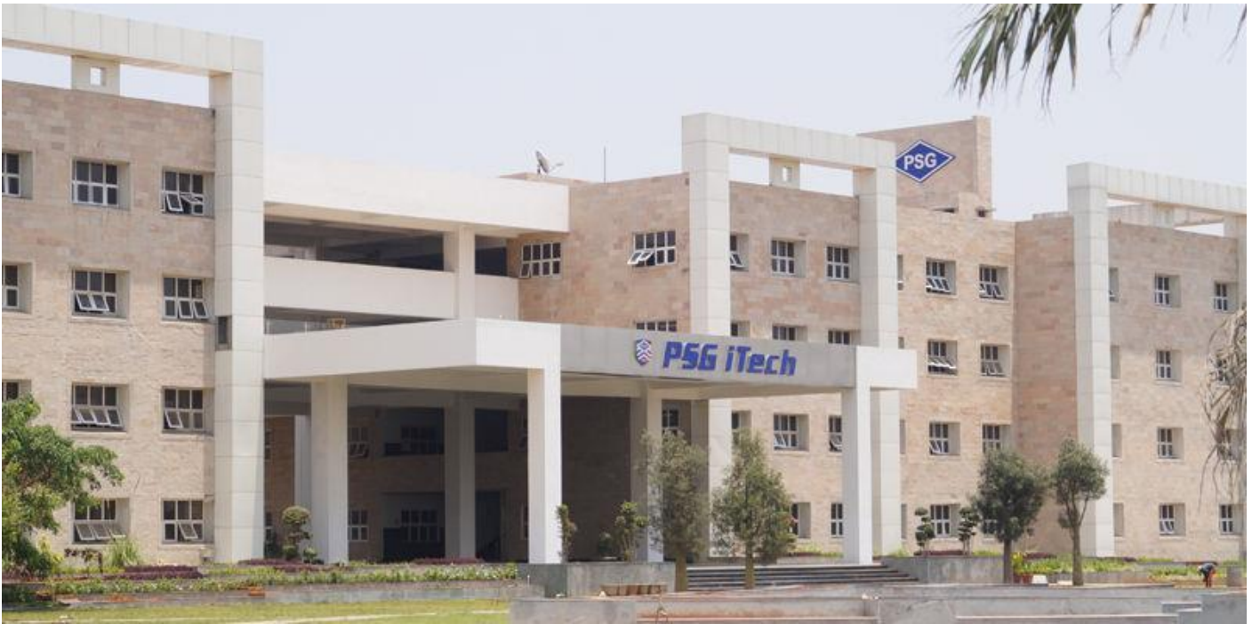
Figure 1: Teaching block buildings showing recessed windows on the North elevation
